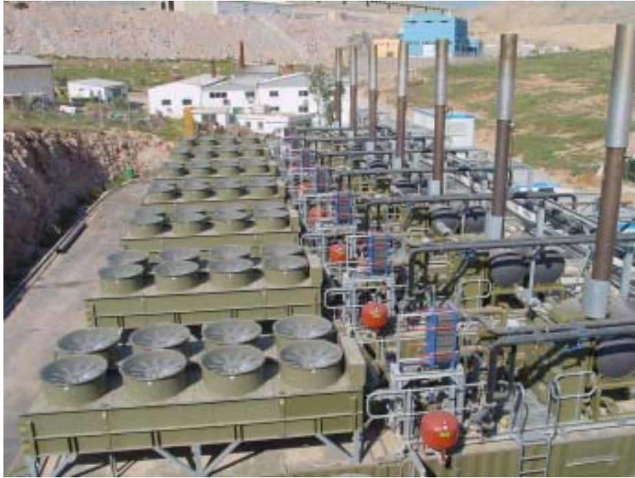
General view of the engines of the Ano Liosia cogeneration plant.
