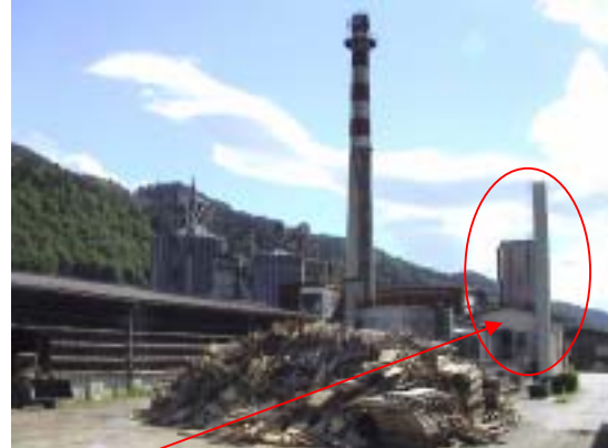
Place for new boiler and steam turbine
