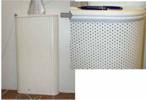
Figure 9 Typical perforated plate wall diffuser
