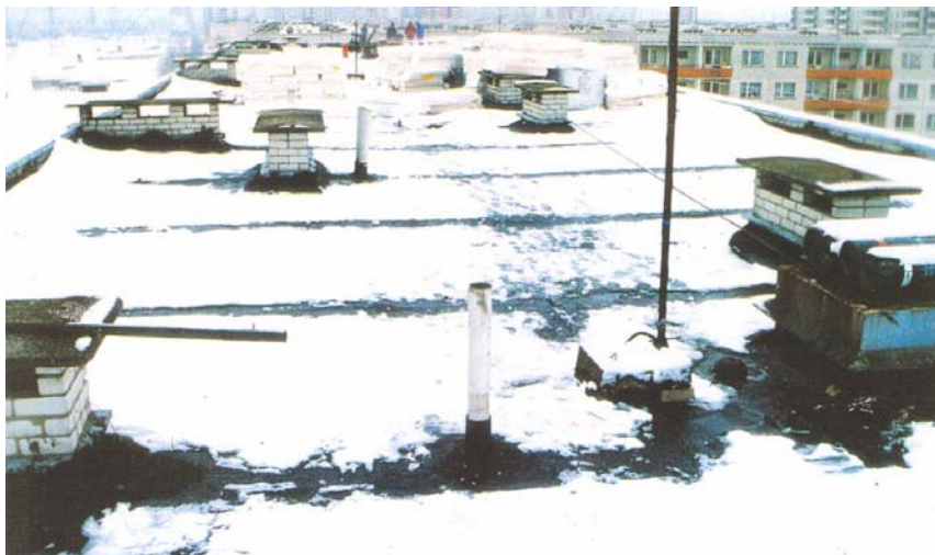
Photo 2 Energy loss through roof
