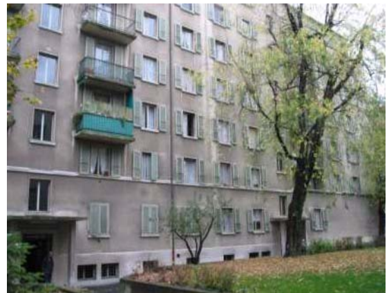
Fig. 4 The building before renovation
