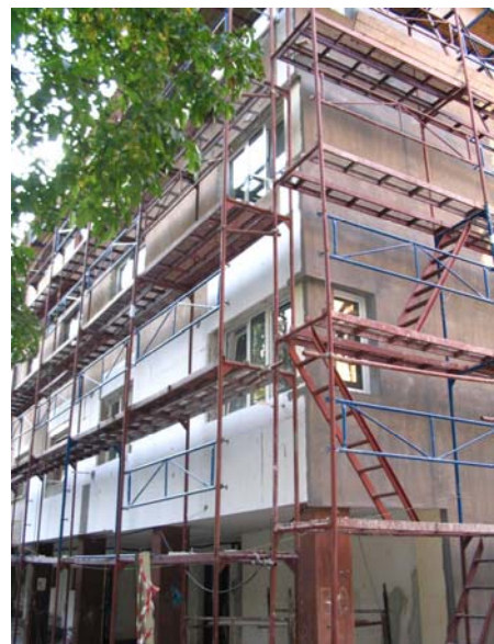
Fig. 3 In process of refurbishment
