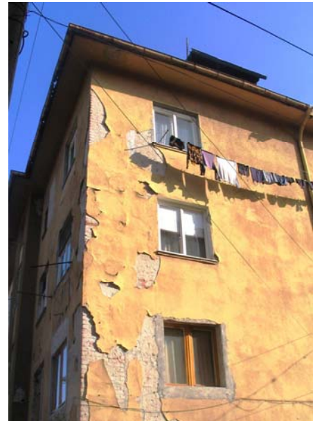
Fig. 1 Building before renovation
