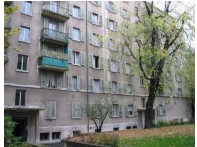
Building before renovation
