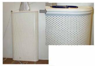
Figure 9 Typical perforated plate wall diffuser
