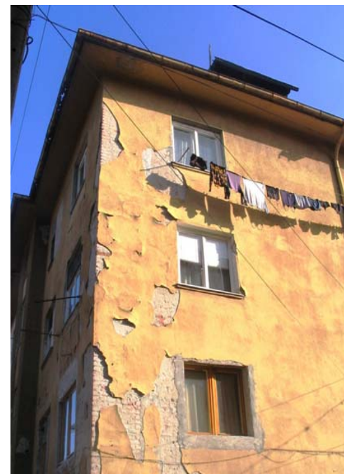
Building before renovation
