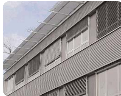
Figure 5 Protection from the sun with horizontal overhangs and external awnings in an office building in Dresden (D)
