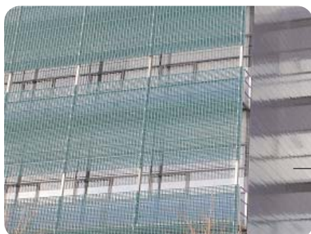
Figure 4 Vertical shadings devices in an office building in Dresden (D)
