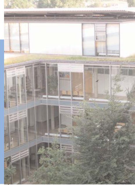
Figure 2 Offices of Chamber of Commerce in Freiburg (D): correct example of application of techniques to reduce summer thermal loads (sun protection and ventilation of roof), shading devices and green roof.
