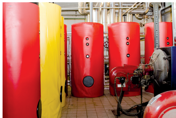
Picture 4: Boiler Room at Red Cross Centre
