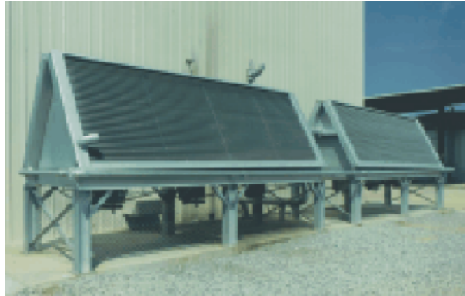
Figure 4.4. The system's air-cooled condensers
