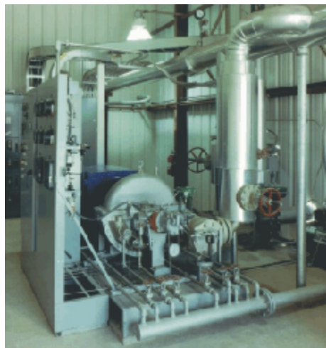
Figure 4.1. The turbine generator installation
