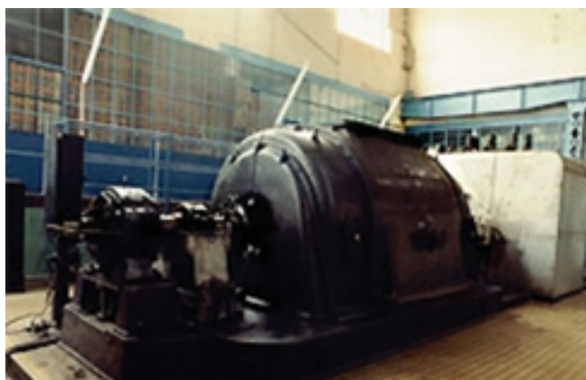
Steam Turbine at CHP Plant Timisoara Centru
