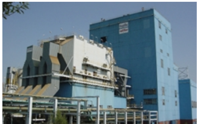
Combined Heat and Power Plant Bielsko-Biała
