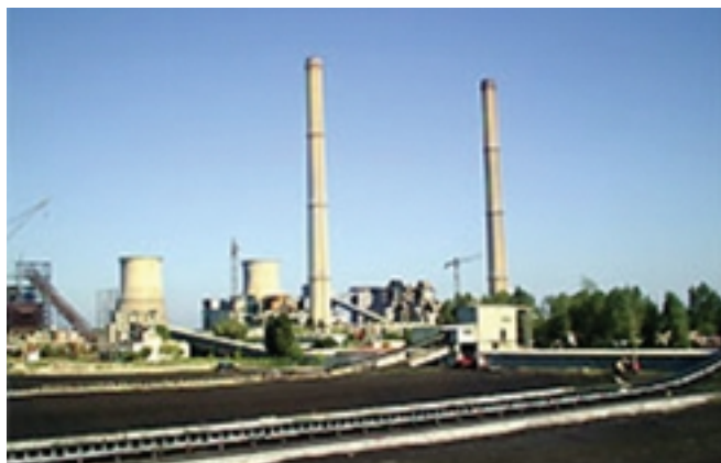
Combined Heat and Power (CHP) Plant Timisoara Sud
