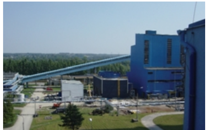
Combined Heat and Power Plant Bielsko-Biała
