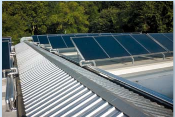
View of the solar collectors on the building's roof.
