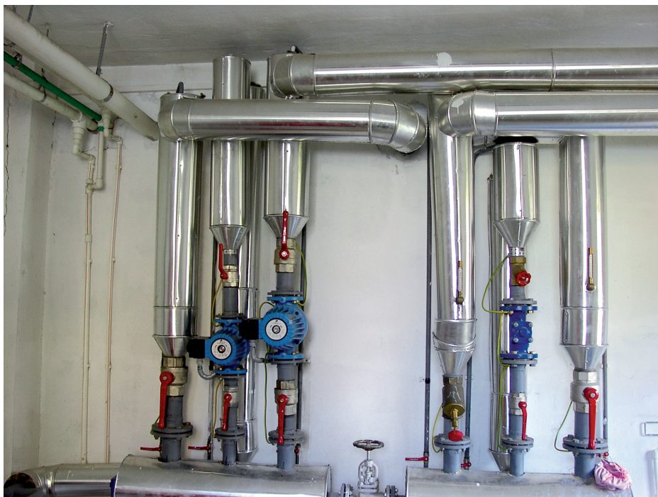
Picture 1: Pipework in boiler room
