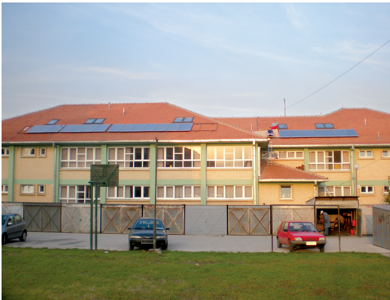
Picture 3: Collector installation
