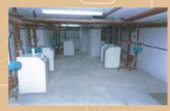
According to measurements made during the first year of operation, COP of the GSHPs for heating and cooling are  $COP_{th}=4$  and  $COP_{c}=3.5$  respectively.
