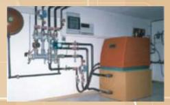
The GSHP system is composed of a supply and a return well. Groundwater flow rate is about 3 m<sup>3</sup>/h.
