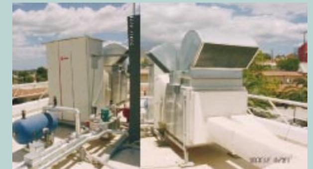
Solar assisted water - air heat pump
