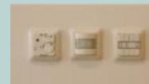
Room thermostat, occupancy sensor, and eight function switch installed throughout the building's rooms
