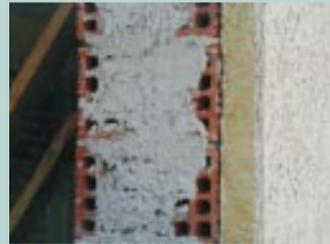
Detail of external brickwork with external insulation
