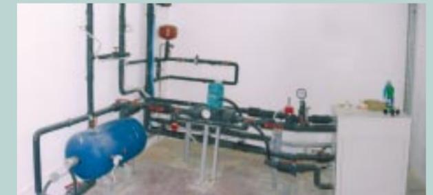
Geothermal water to water heat pump
