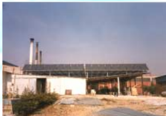
Solar collectors on roof
