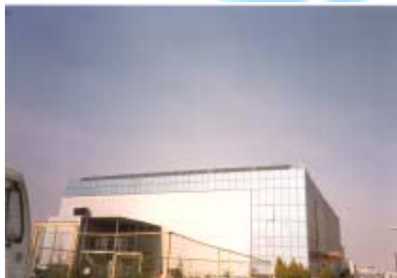
Solar collectors on roof
