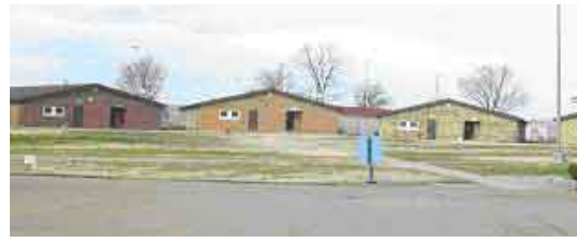
Fig. 1. Guilds 5, 6, and 7 at NWCX . Guild 5 is on the left, 6 is in the middle, and 7 is on the right.
