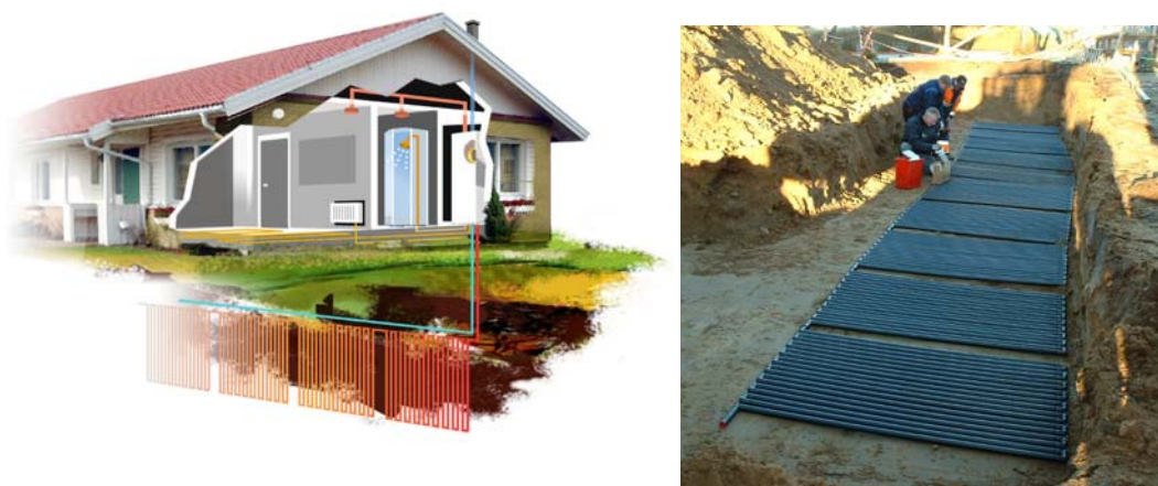
Fig. 8. Vertical and horizontal installation
