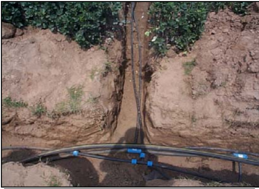
Details of Earth Loop
