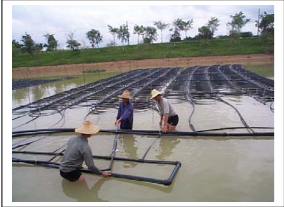
Laying Loop Piping
