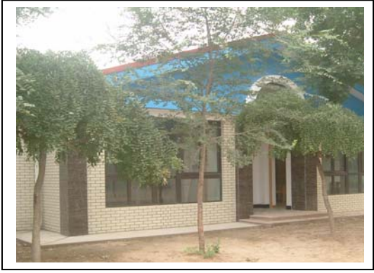
One School Kindergarten Building
