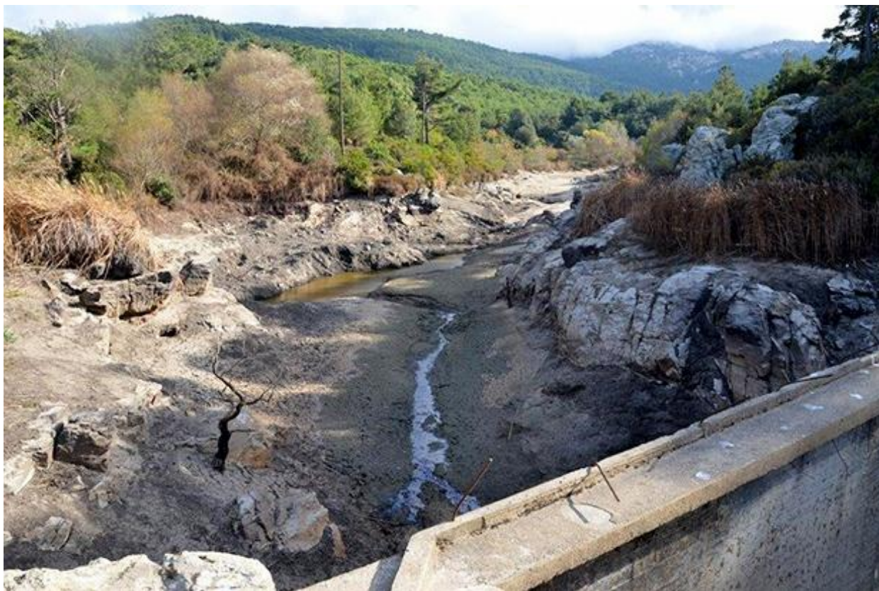
EMPTY WATER RESERVOIRS
