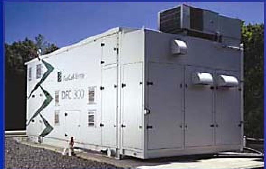
Fuel Cell Energy's 250 kW MCFC
