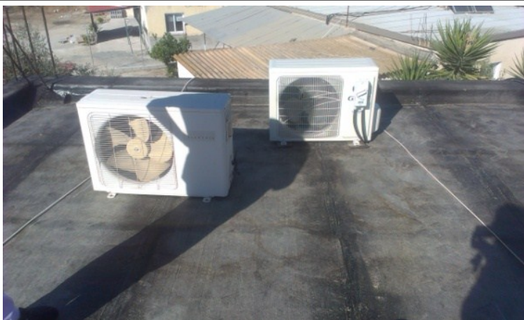
PP1 – Waterproof insulation and new a/c units
