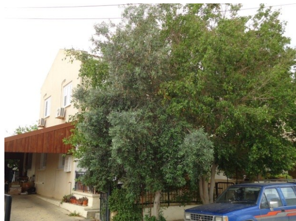
PP25 – Before works
