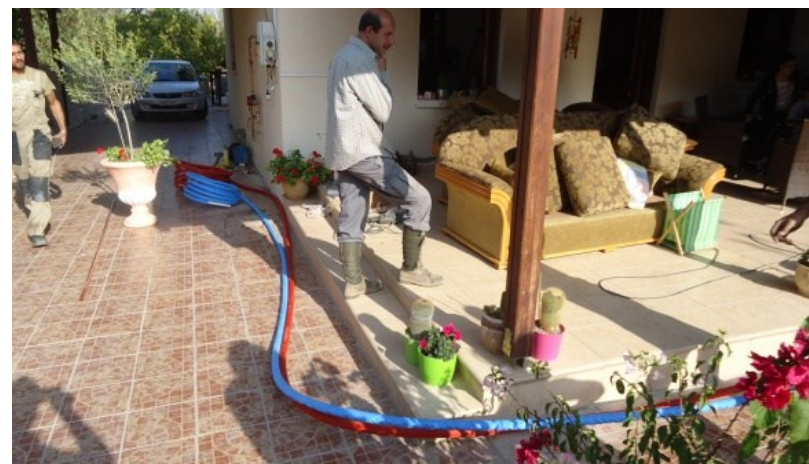
PP8 – Piping workings for the installation of the fireplace
