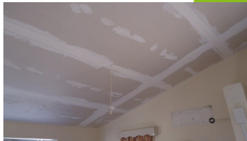
PP15 – Ceiling with thermal insulation
