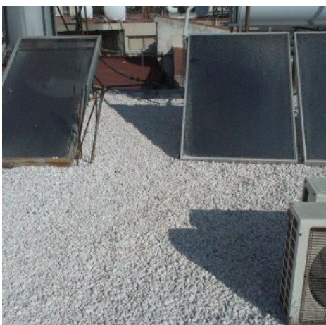
PP12 – Thermal Insulation of the roof
