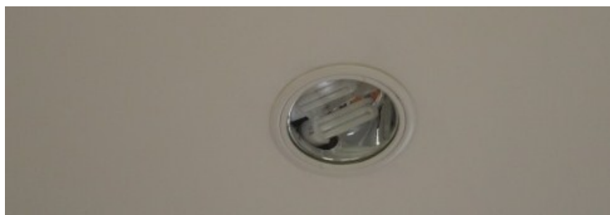
PP7- Efficient lighting and new ceiling with thermal insulation
