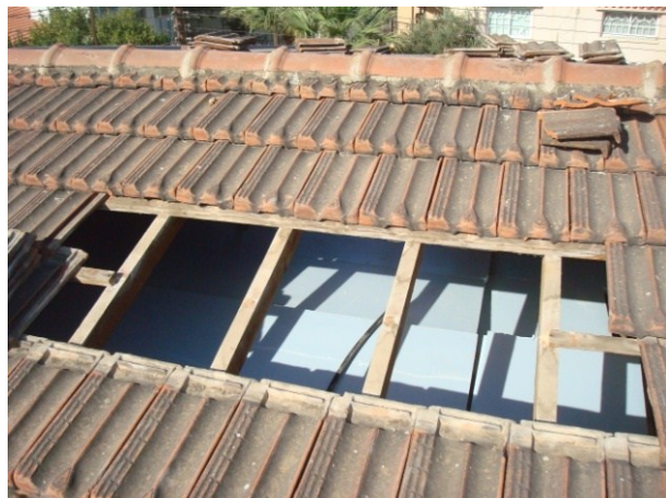
PP16 – Thermal Insulation of the roof
