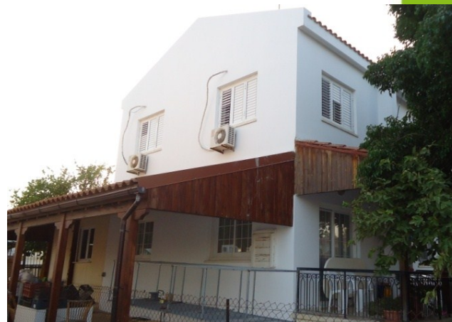
PP25 – After thermal plaster
