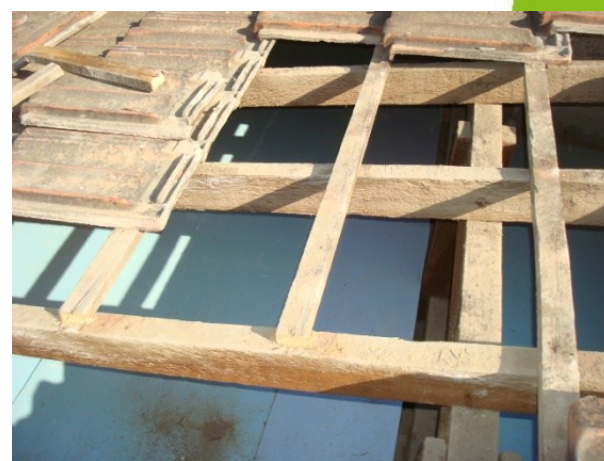
PP16 - Thermal Insulation of the roof
