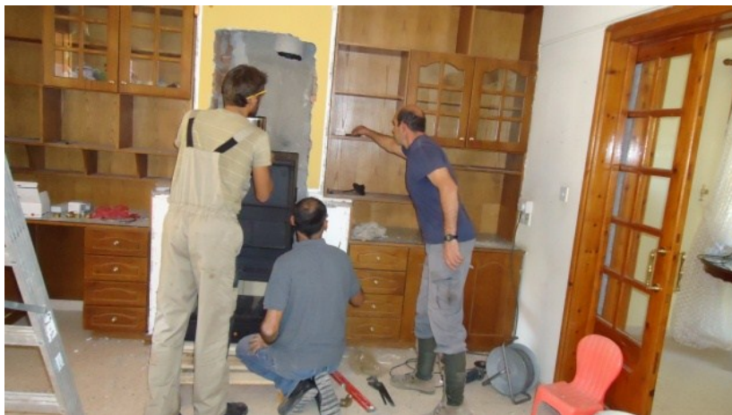
PP8 – Efficient fireplace (with boiler) installation
