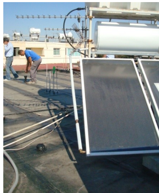
PP4 – Waterproof Insulation and new solar thermal water heater
