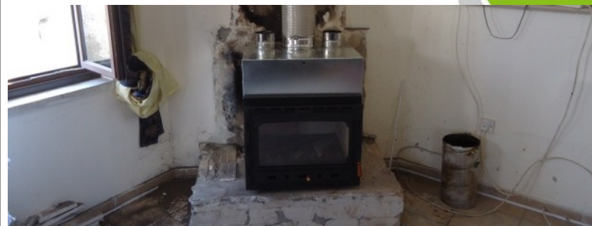
PP7- New efficient fireplace (air module)
