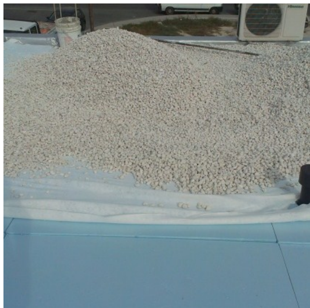
PP4 – Thermal Insulation of the roof
