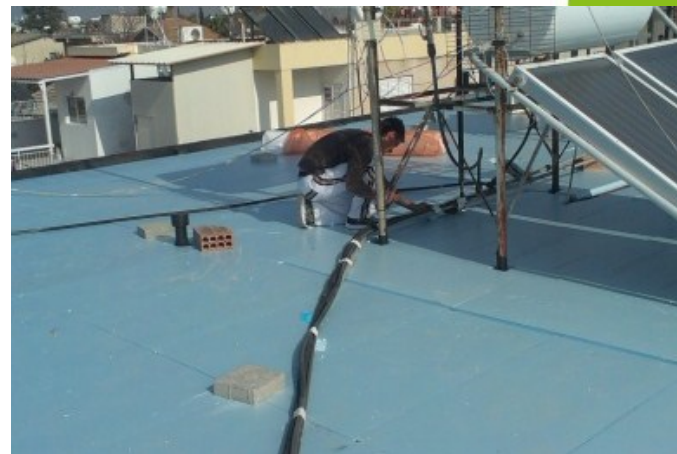
PP2 – Thermal insulation and new solar thermal water heater
