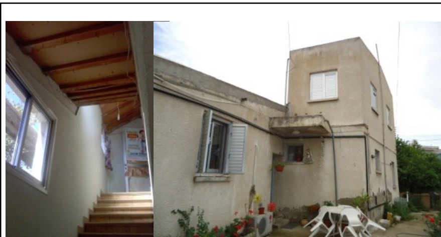
PP13 – Indoor and outdoor before
