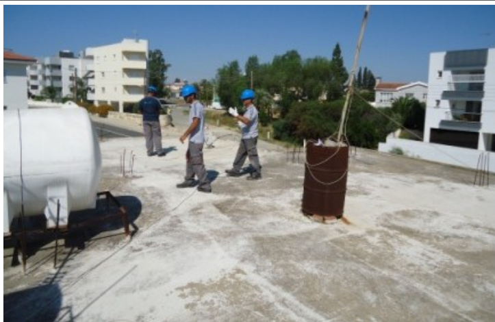
PP20 – Roof before insulation
