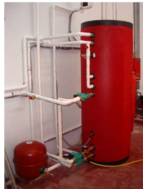
Hot Water Storage Tank, 500l
