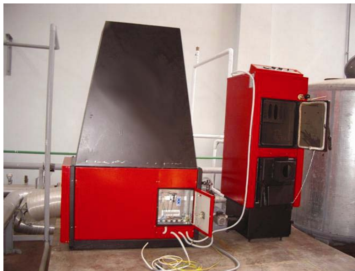
Biomass Boiler, 35kW
