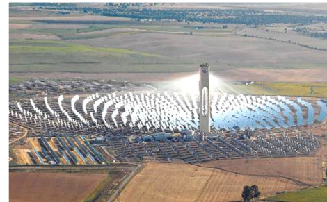
10 MW STE plant co-located with 1 MW PV in the Solucar complex, Seville, Spain
