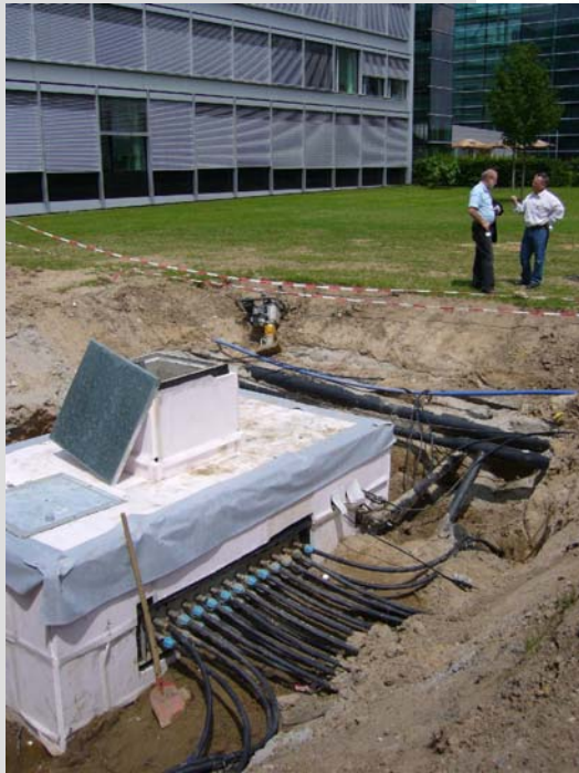
BHE-field, manifolds and pipes in the building
