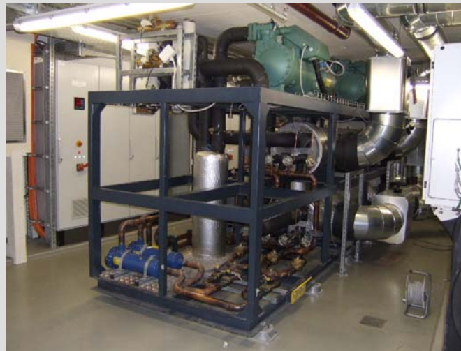
Heat pump and groundwater heat exchanger
