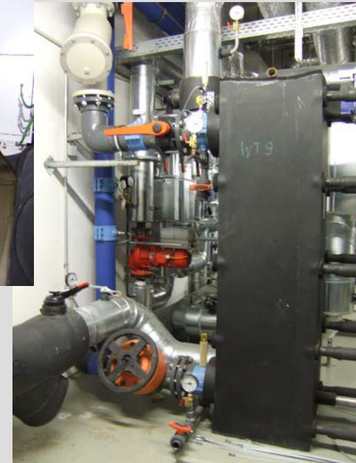
Heat pump and groundwater heat exchanger
