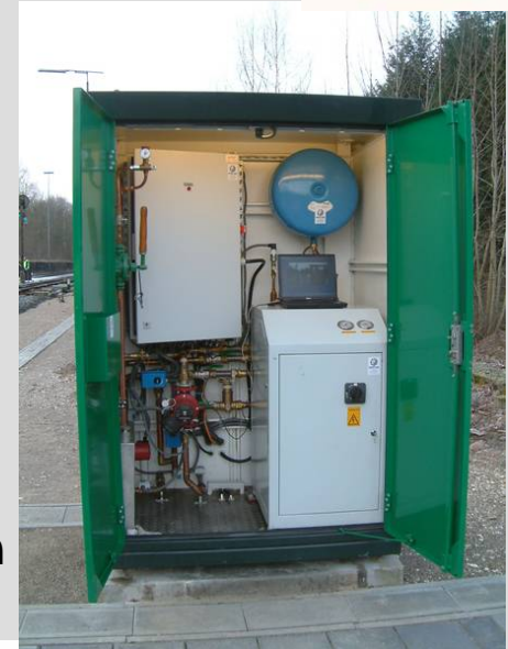
Heat pump installation (right)
