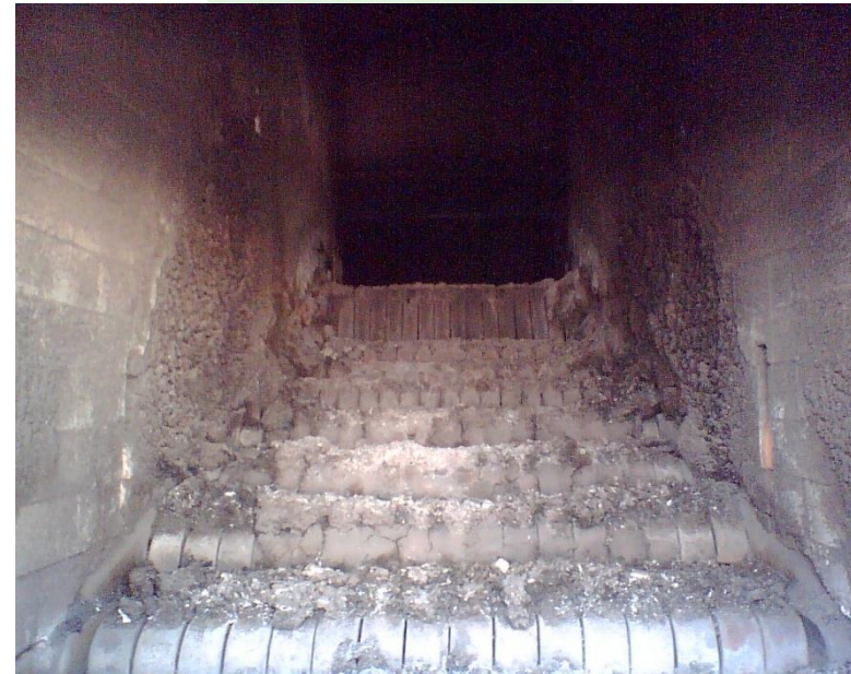
Slagging of the combustion chamber walls by the use of inferior fuel
