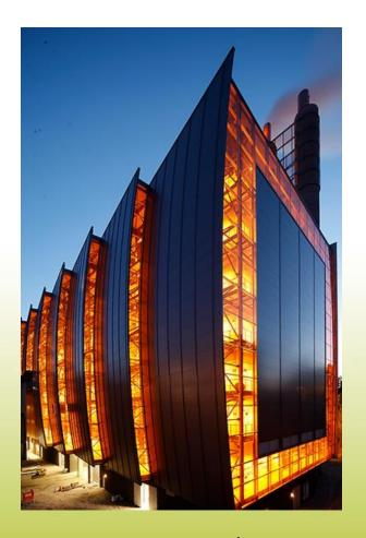
Incineration of burnable waste - 410 000 tons/year. Production of hot water for district heating (840 GWh) and electrical energy (160 GWh)
