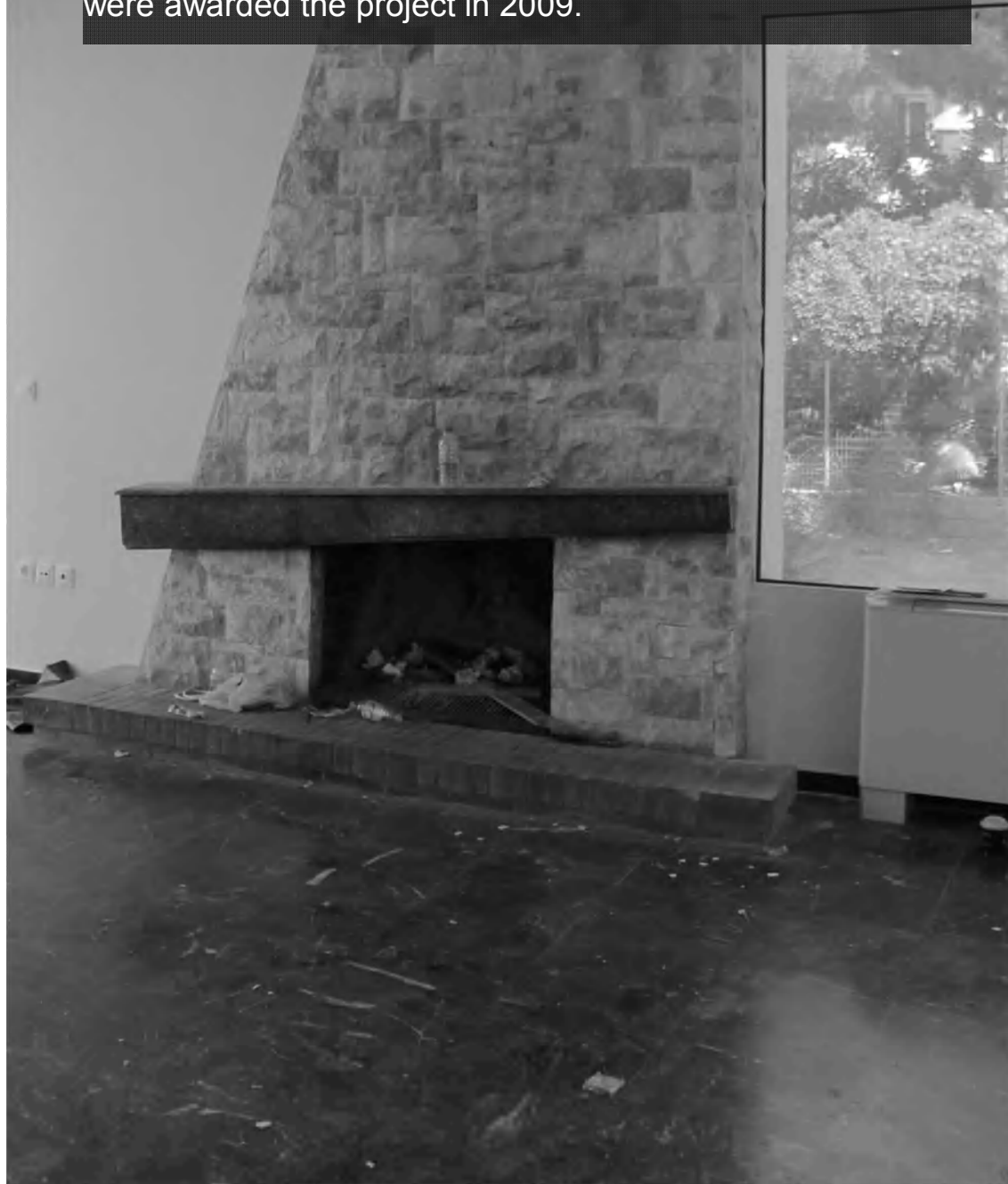
pre-existing fire place
