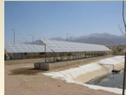
Jordan, 2005 BWRO 3.41 m 3 /h, 16.8 kWp PV
