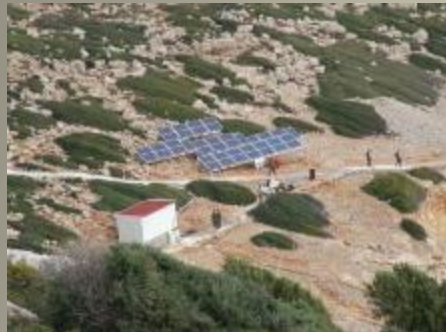
Strogili island, Greece, 2012 SWRO 0,33 m 3 /h, 20 kWp PV
