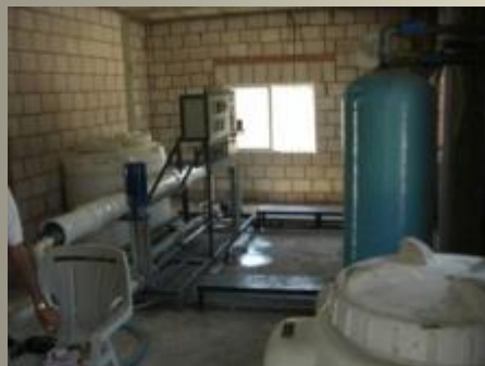
Jordan, 2010 BWRO 0.83 m 3 /h, 10.4 kWp PV
