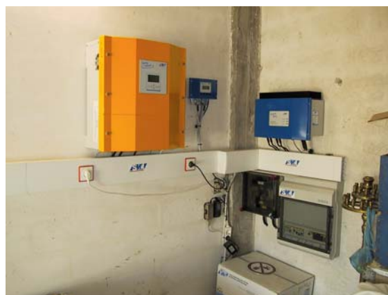
Fig. 4. A view of the PV system power electronic hardware located inside the farmer's house.
