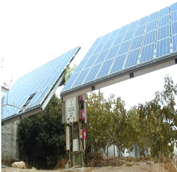
Figure 4: Photovoltaic array of 4.4kW p
