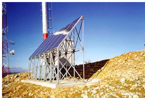
Figure 4: A 2.4kWp PV system for a repeater station at mountain Dirfi, central Evia
