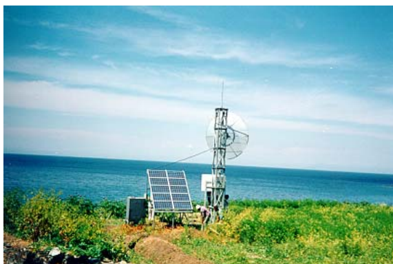
Figure 3: A typical solar-electrified outstation at the Holy Mountain
