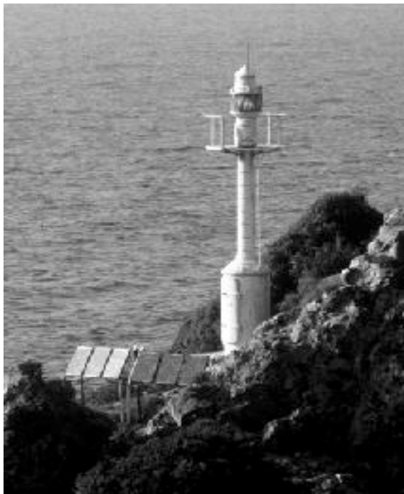
Figure 2: Stand-alone PV powered navigational aid.
