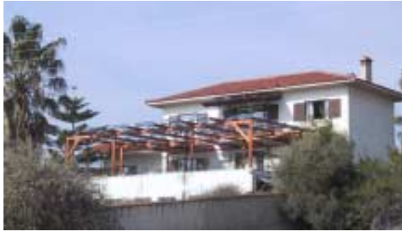
Fig. 4 CRES-3 pergola PV system at the main building
