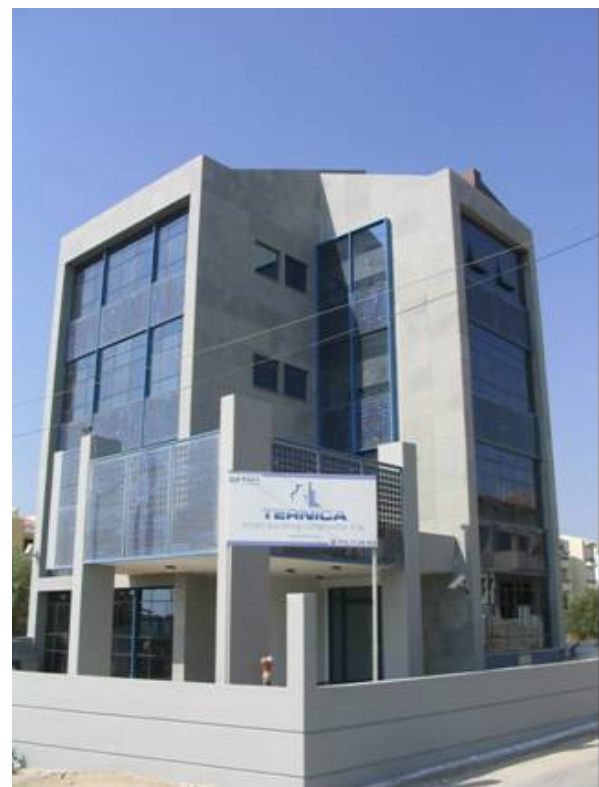
Figure 7: An office building in Maroussi, Greece with a 11kWp BIPV system.
