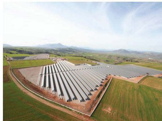
Figure 2: Two PV systems 2MWp and 1,25 MWp, of the same owner, installed one next to the other near Thiva.
