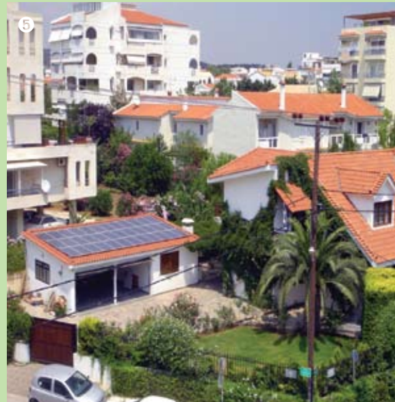
A Photovoltaic system of 6KW power in domestic house at Voula region in Athens city Source: Data energy
