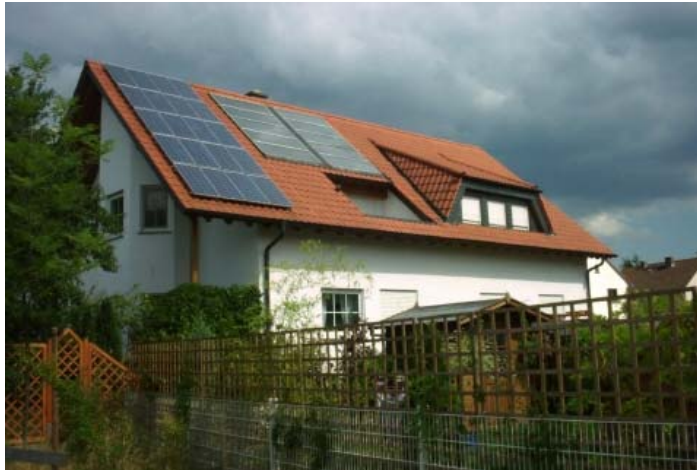
Solar PV roof in residential building
