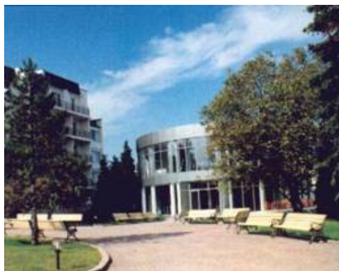
Hotel Bankya Palace-general view
