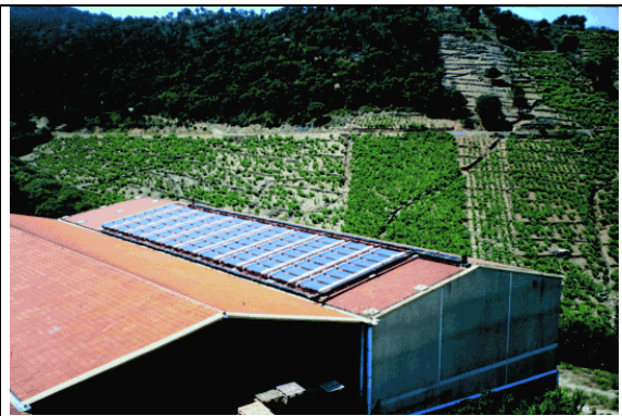
Figure 4.5: Solar cooling of a wine cellar in Banyuls, France (source: IEA Task 25)
