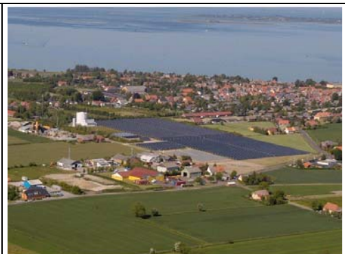
Figure 4.3: Solar district heating in Denmark (source: Marstal Fjernvarme Amba)
