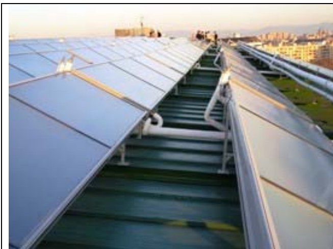
Figure 1. Solar collector modules (58 units of 5,8 square
