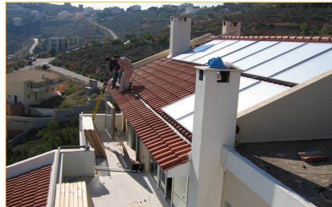
collector with transparent heat insulation
