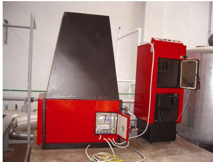
Biomass burner, 35kW
