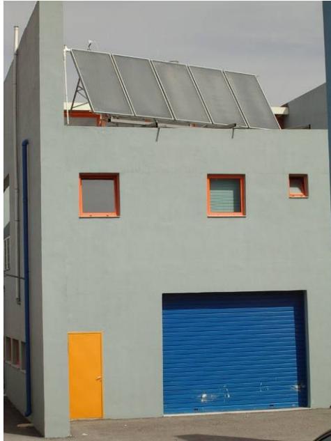
Heated Offices, 60m 2
