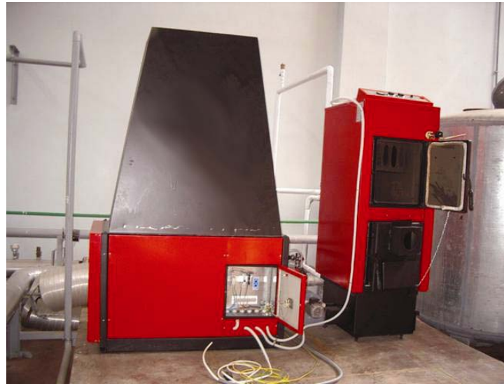
Biomass burner, 35kW
