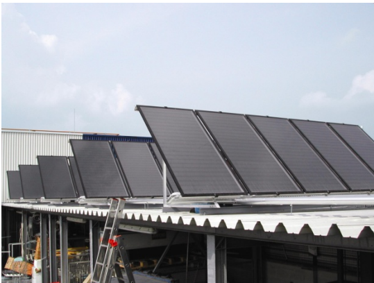
Tesco department store, Érd
