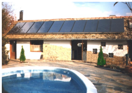
Swimming pool heating
