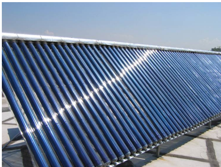
Figure 12: Vacuum-tube collectors installed in Iberostar Hotel, Sunny Beach, BulgariaHotel
