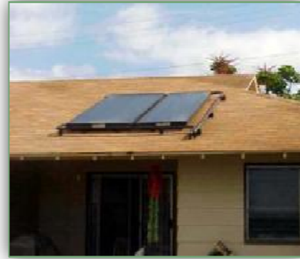
picture 2: Typical DHW system for a single family house (Source: FME-Diploma work)
